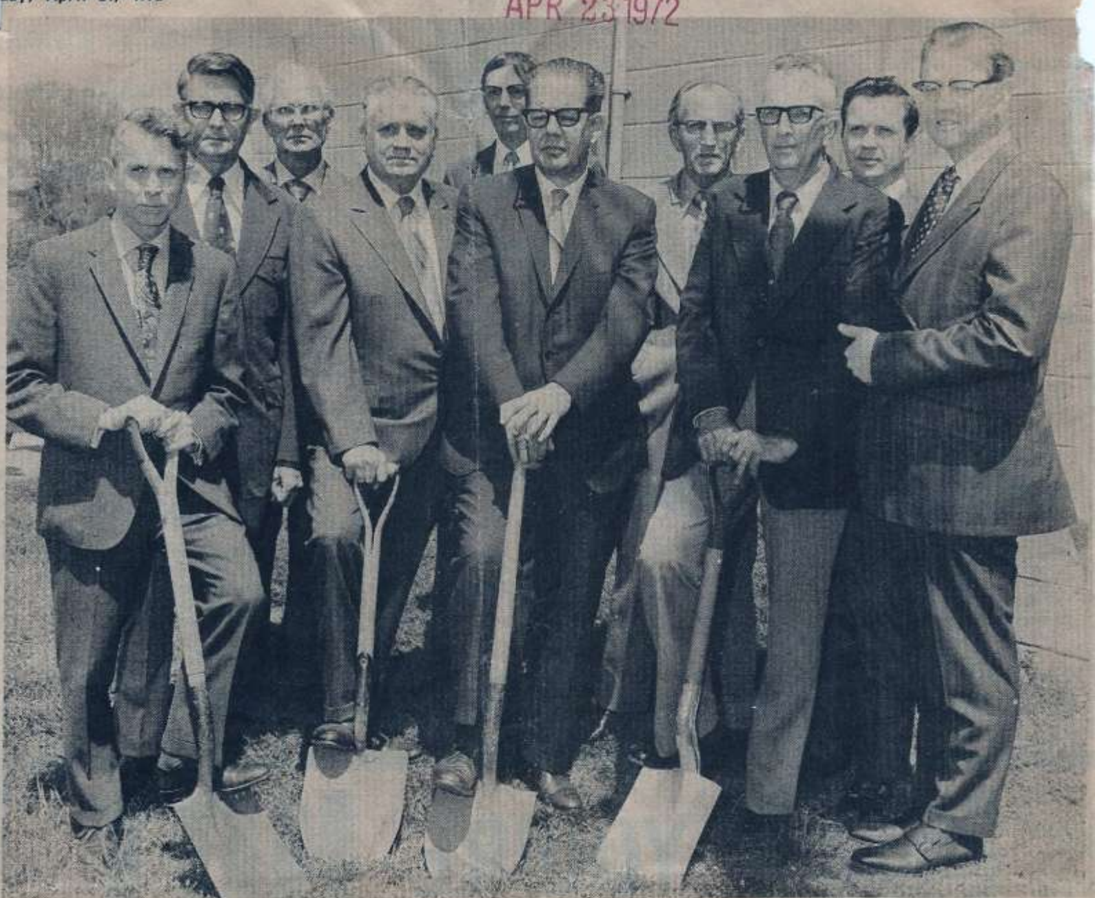
BREAKING THE GROUND for a new $150,000 educational building at Graymere Church of Christ are (left to right, front row) James Farris, Elder; Lloyd Pruett, elder; Vernon Gilliam, elder; Arden Eskew, Dr. Batsell Barrett Baxter; (back row) J. C.
